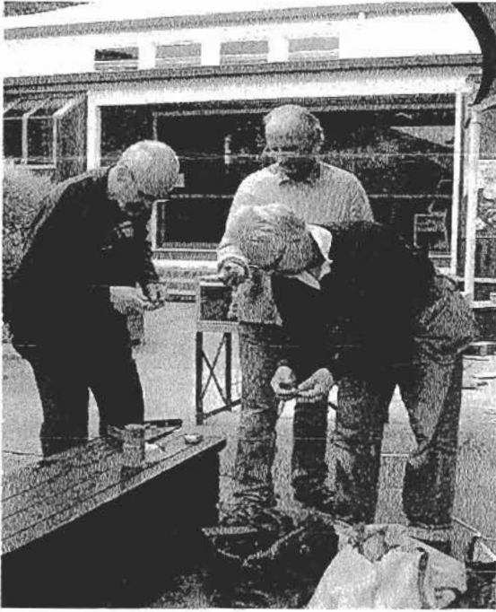
Three familiar faces at a working bee one day in January to build a new and permanent outdoor stage in courtyard of Muritai School .
